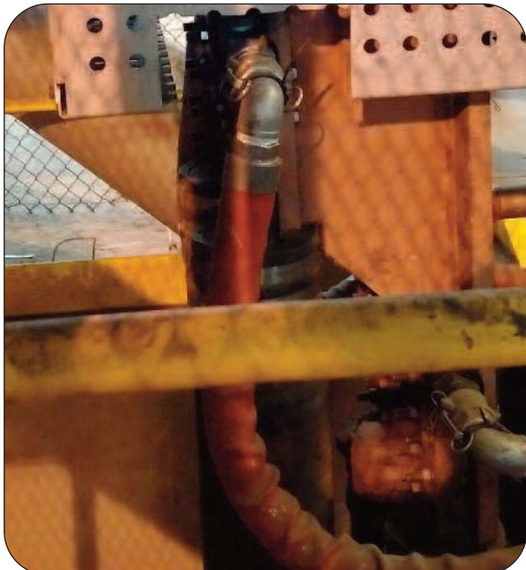
Thorburn's 48TSP-NC Furnace Door Hose Assembly with Cam-Lock Model 733 DBW Butt Weld Quick Coupling System installed at a Pyrometallurgical Nickel Smelter transferring dissolved chlorides
